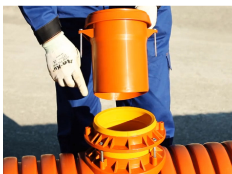
8 Inserimento codolo 8 Application of socket
