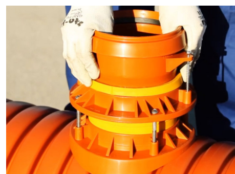
9 Serraggio viti autofilettanti 9 Tightning of self-tapping screws
